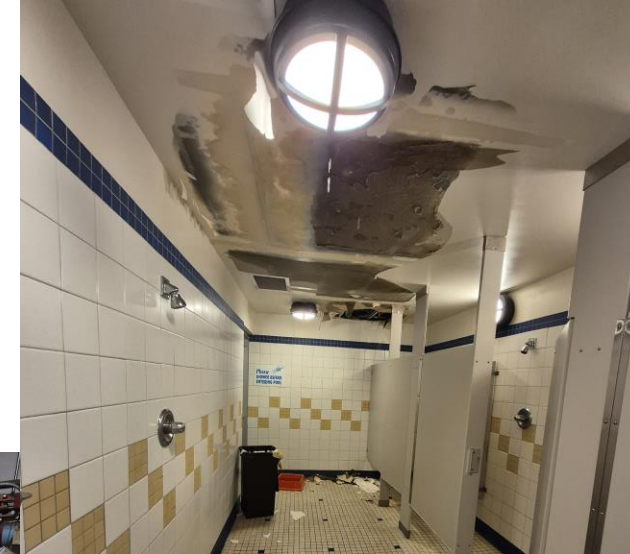
Above – Water damage from plumbing failures
