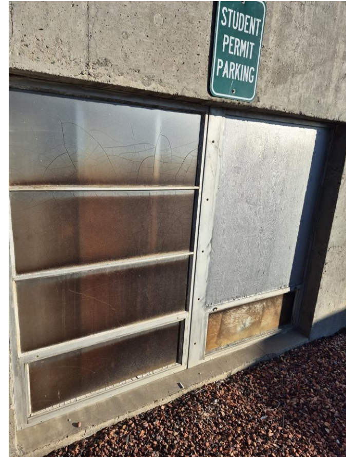
Typical deteriorated window condition
