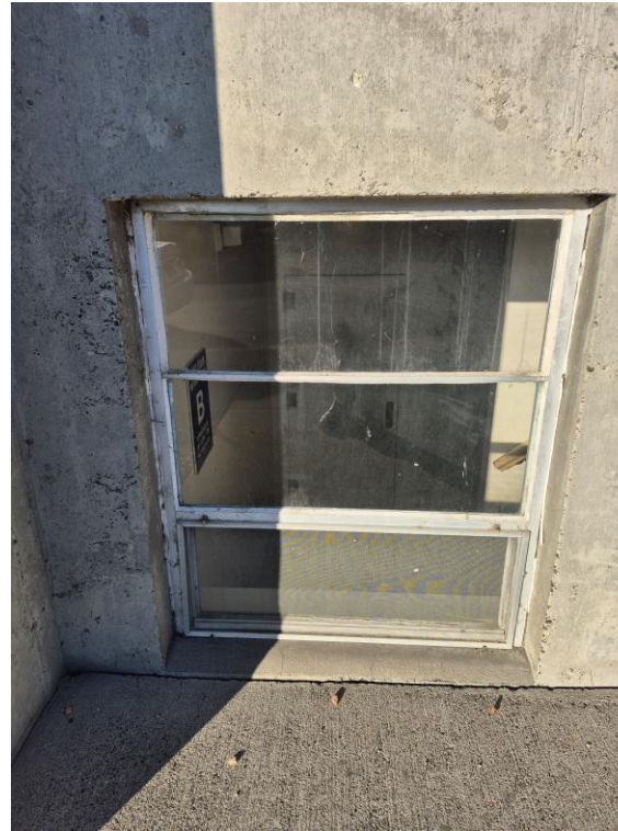
Typical deteriorated window condition
