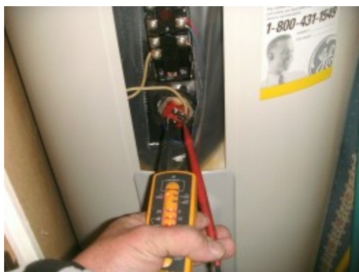
Voltmeter in use - know what voltage you will be dealing with, and if it is hot.
